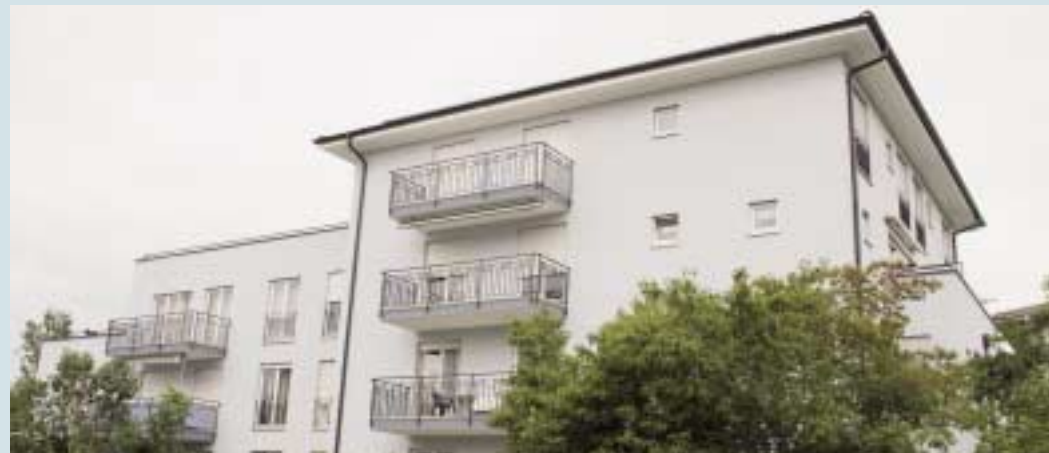
Dieselstraße 61/61a, Ettlingen
